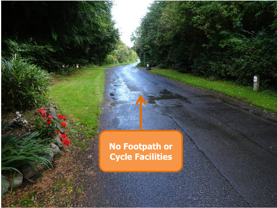
Figure 2.2: Lack of Footpath Facilities along Local road L5078
